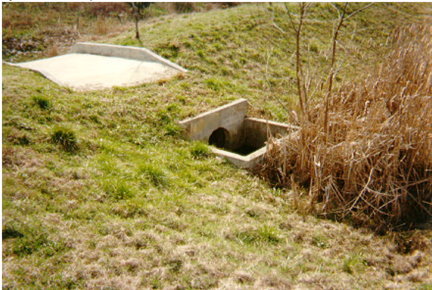
Photo 3: Outlet structure, showing cattails partially blocking the 22 in orifices through concrete wall (photo by John Easton).
